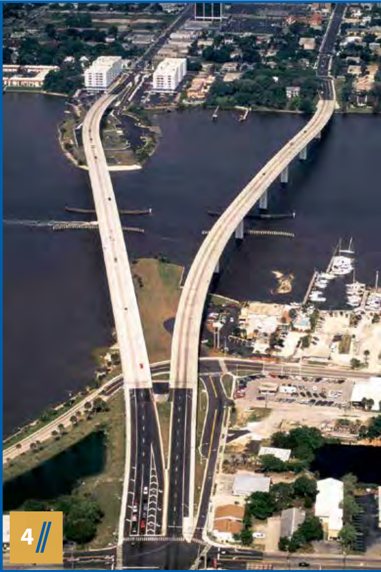
4 // Seabreeze Segmental Bridge Daytona Beach, FL
