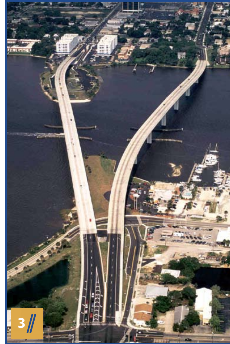
3 // Seabreeze Segmental Bridge Daytona Beach, FL
